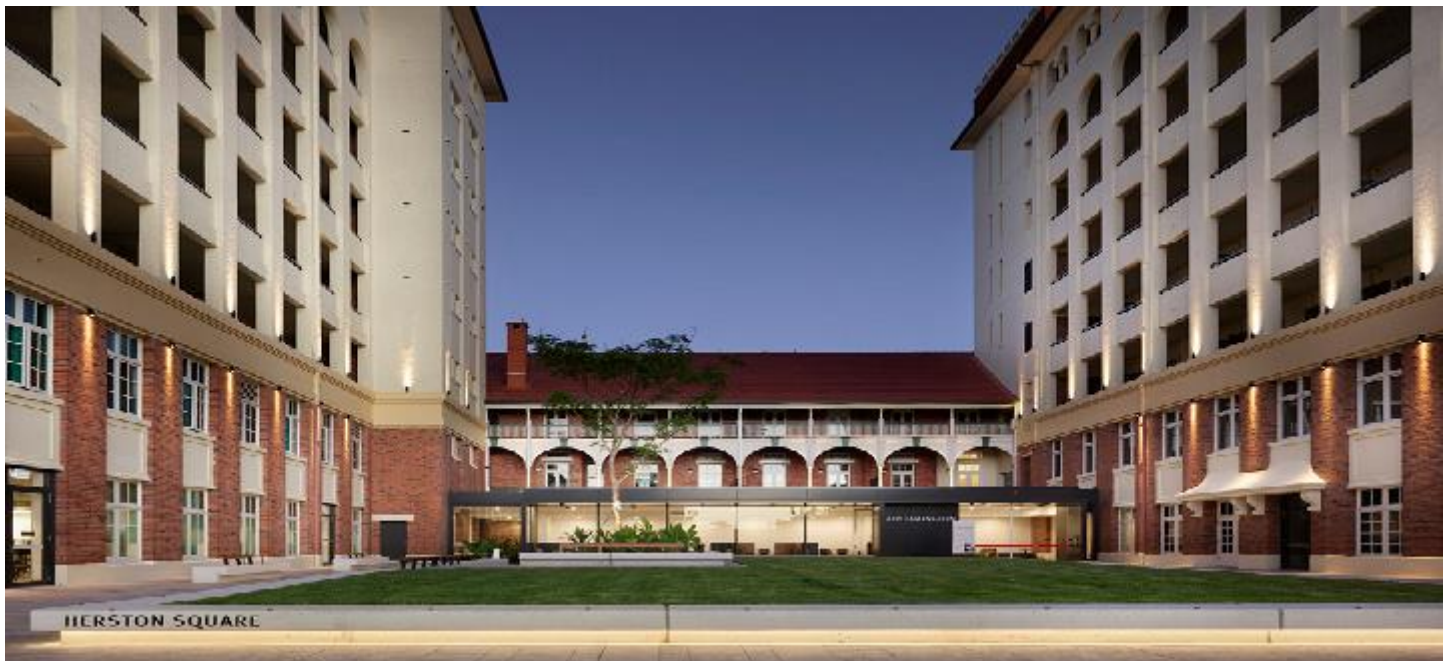
Australian Unity Student Accommodation Fund, Lady Lamington Building, Herston QLD (Photo Credit: Scott Burrows)
