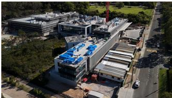
Wyvern Private Hospital (under construction), Terrey Hills, NSW
