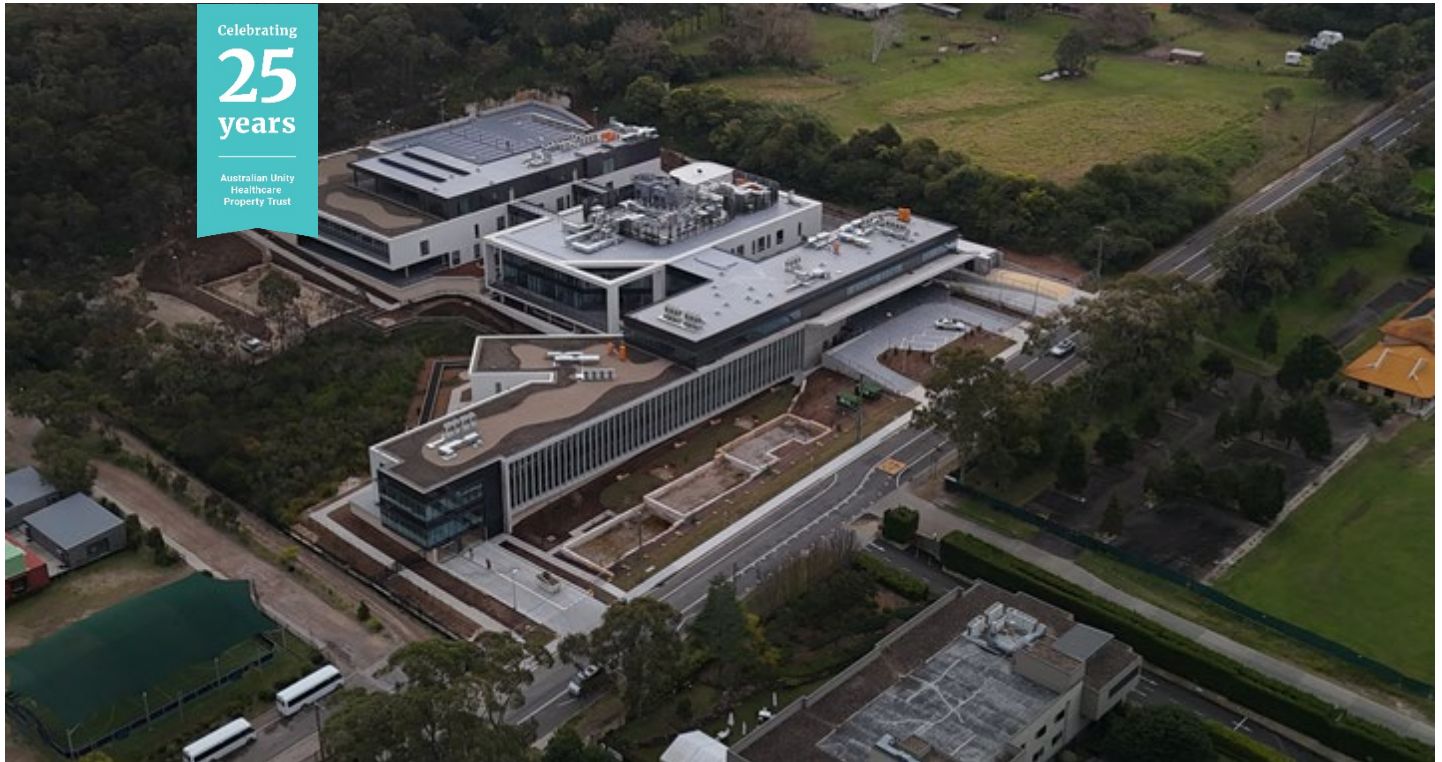
Wyvern Private Hospital, Terrey Hills, NSW
