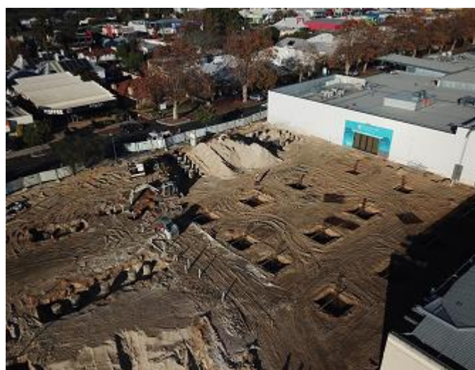
Busselton Central Shopping Centre Stage 3, Busselton, WA
