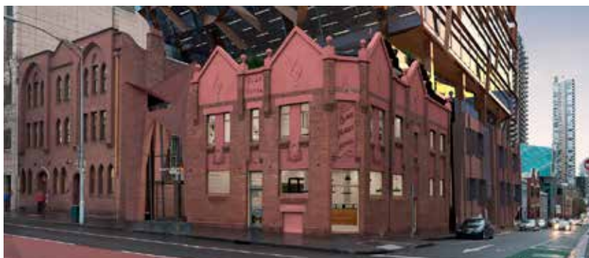
Australian Unity Head Office, 271 Spring Street, Melbourne
